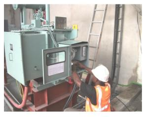
This involves physical check-up and testing of existing system to ascertain its electrical soundness and give recommendations for further steps to be taken.
